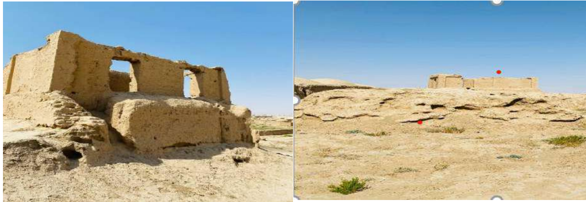
Figure.1. Interior & exterior picture of the old castle
